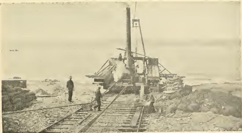
REAR VIEW OF CAPE NOME HYDRAULIC MINING CO.'S BEACH MACHINE, SHOWING SLUICE BOXES, PILES OF COAL, AND TRACK ON WHICH MACHINE RAN OUT INTO THE WATER.
